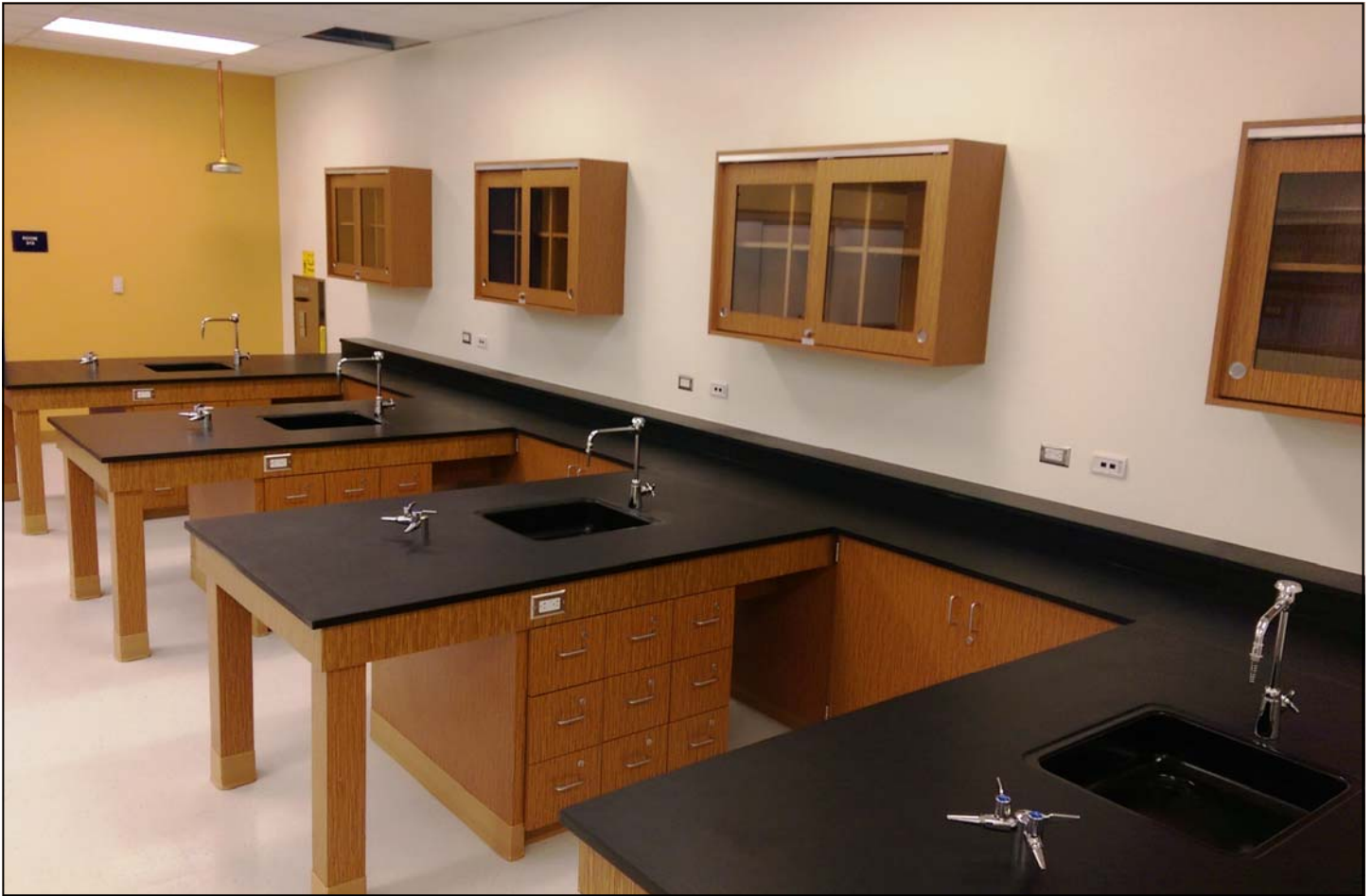
Gas, water, air supply and fume hood were installed into science rooms, as well as a prep room.
